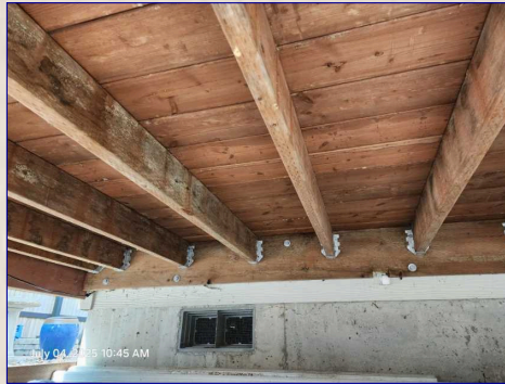
The Joist View
