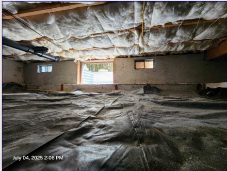
The Crawlspace View
