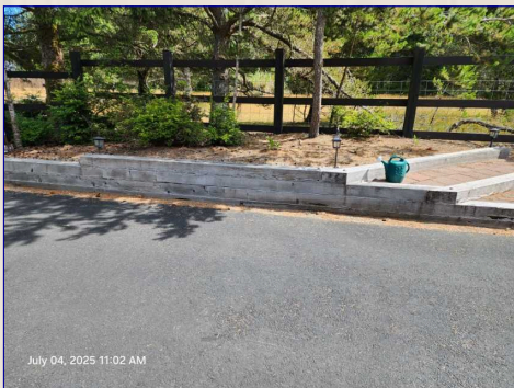
The Retaining Wall View
