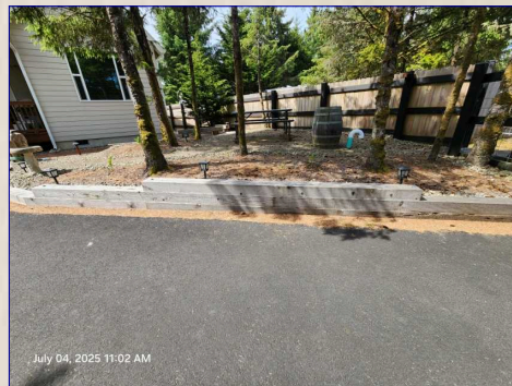
The Retaining Wall View
