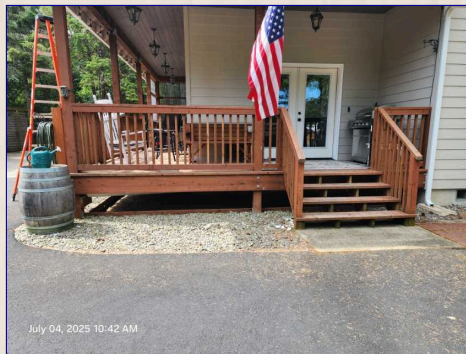
The Deck/Balcony View
