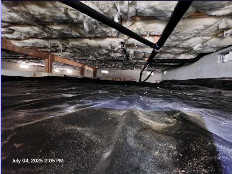
The Crawlspace View
