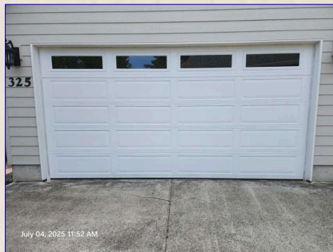
Garage overhead door view.
