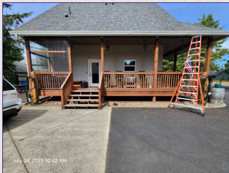
The Deck/Balcony View
