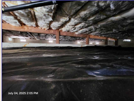
The Crawlspace View
